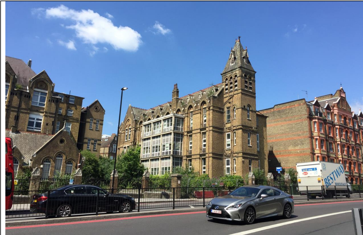
Figure 12: The Charterhouse wing building, looking north west from Archway Road
