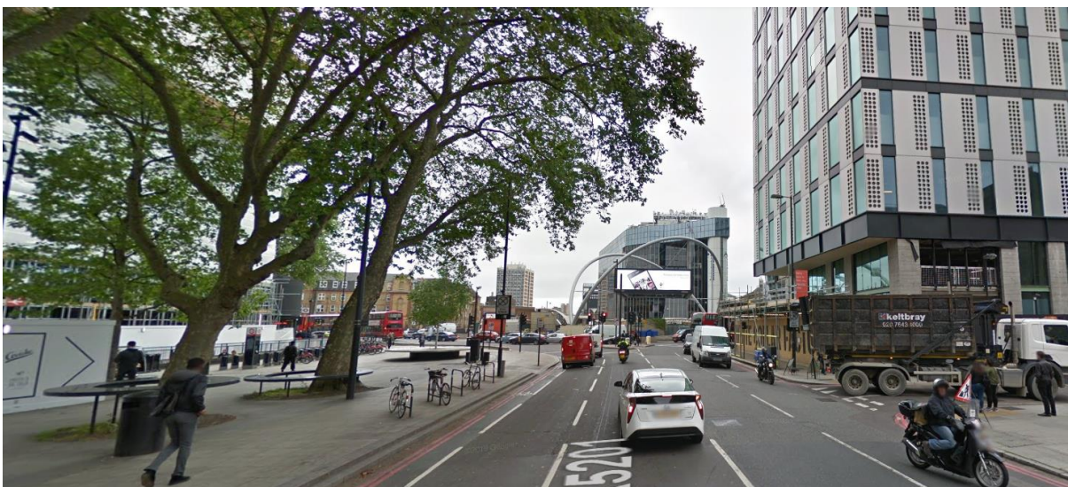
Figure 6: Inmarsat House, viewed from Page 22 along Old Street (prior to roadworks)
