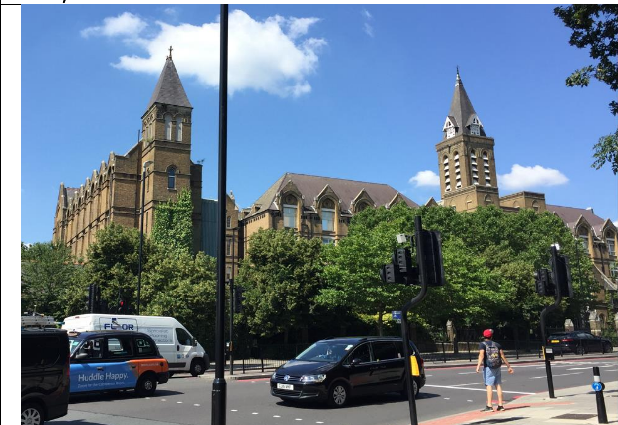
Figure 15: Holborn Union Main Range and Clerkenwell wing building, looking north west from Archway Road
