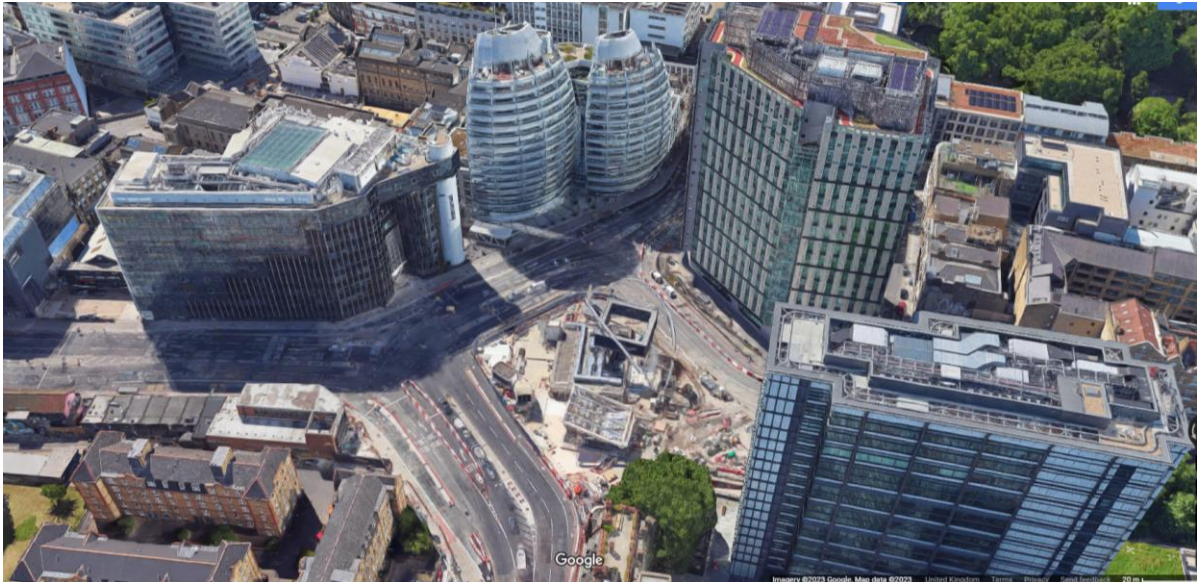
Figure 4: Old Street roundabout with Inmarsat House (L), Bezier (C) and White Collar Factory (R).
